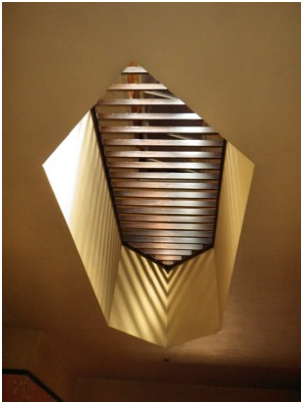
The ingenious air flow/skylight system, viewed from downstairs at left and from upstairs at right, was designed to make the most of the electric heating system
