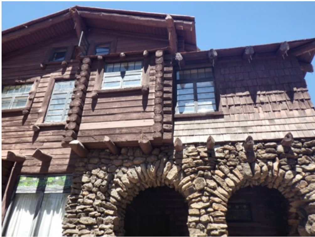
The stone gateway in front of the Mansion; the above photo shows some of the materials used in construction: logs, shingles and stonework
